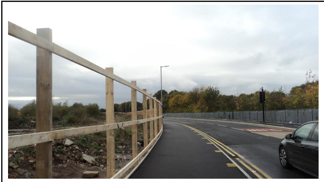
Photo 6 – looking along northern boundary of the site from north eastern corner
